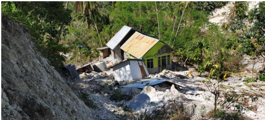
13 housing units in Betania-Nefo Congregation, West Amarasi Presbytery will be relocated because they were destroyed by landslides.
